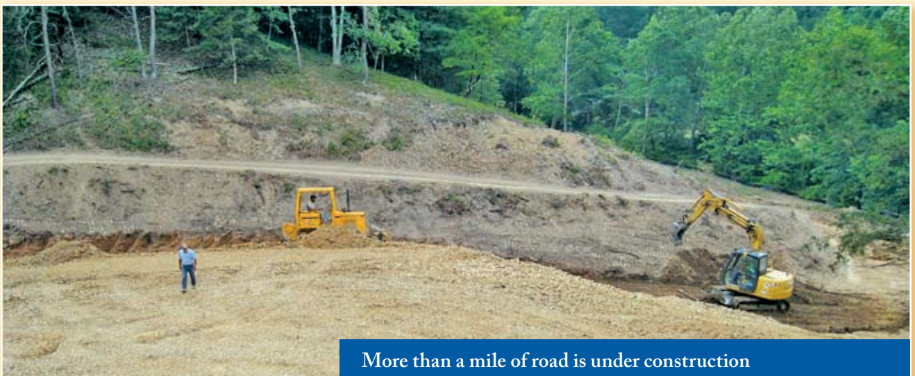
18 acres of timber have been cleared for the road and buildings
